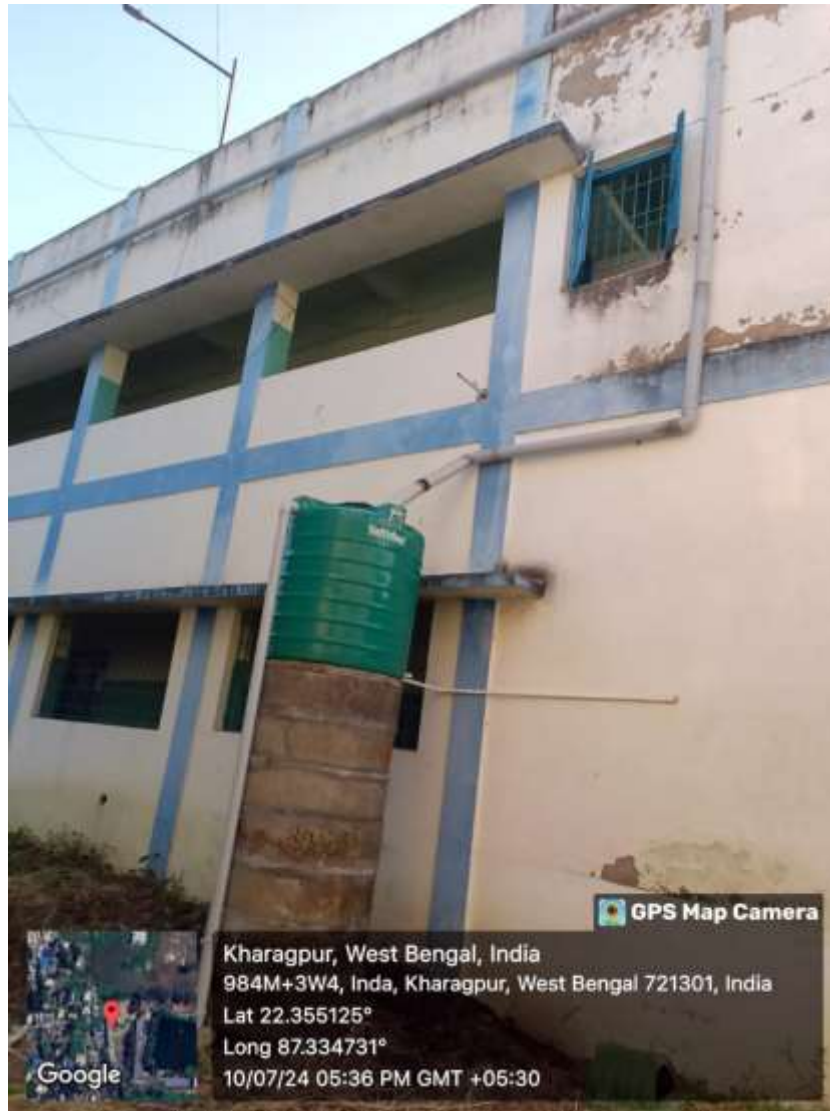
Photograph of Rain water harvesting unit of Kharagpur College
